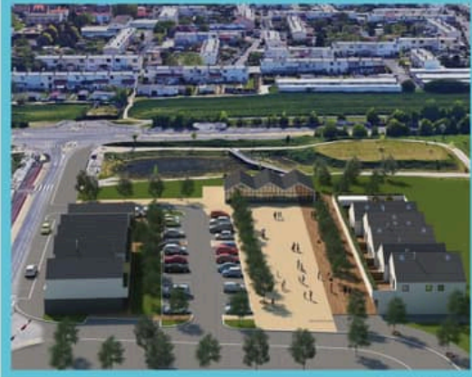
GFS Habitat Construction
